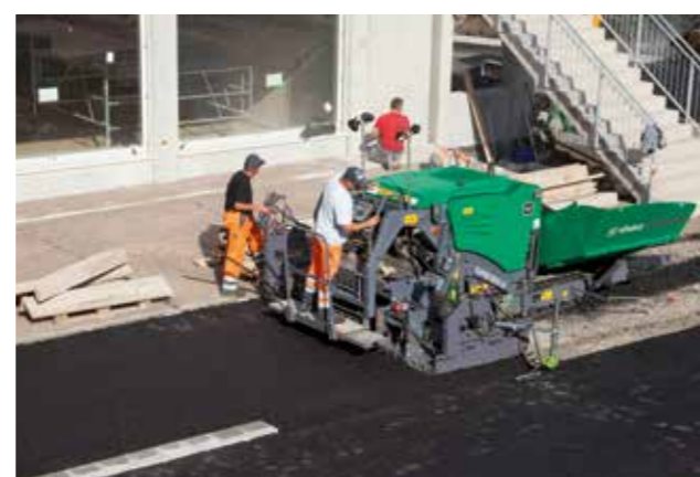
SURFACING LARGE AREAS
