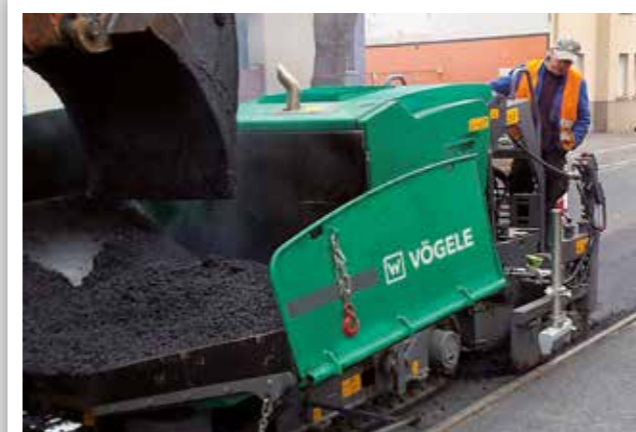
PAVING ASPHALT BETWEEN TRAMWAY TRACKS
