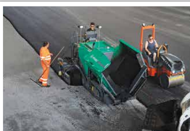
PAVING WORK IN SPORTS FACILITIES
