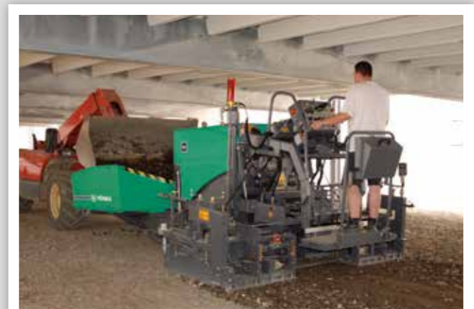
BUILDING THE BASE FOR PAVING SETTS
